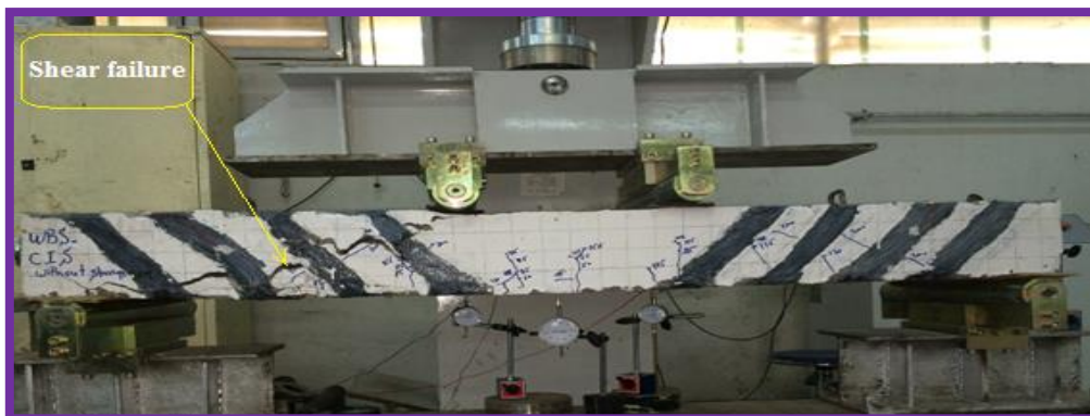
Figure 15: Failure of concrete for (WBS-CIS)
