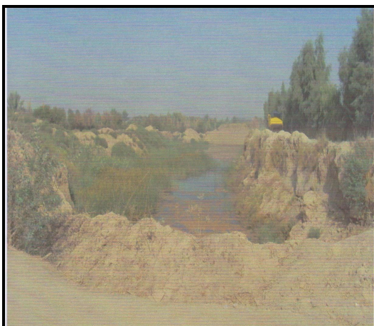
c- Pool of water after excavation with flood plain
