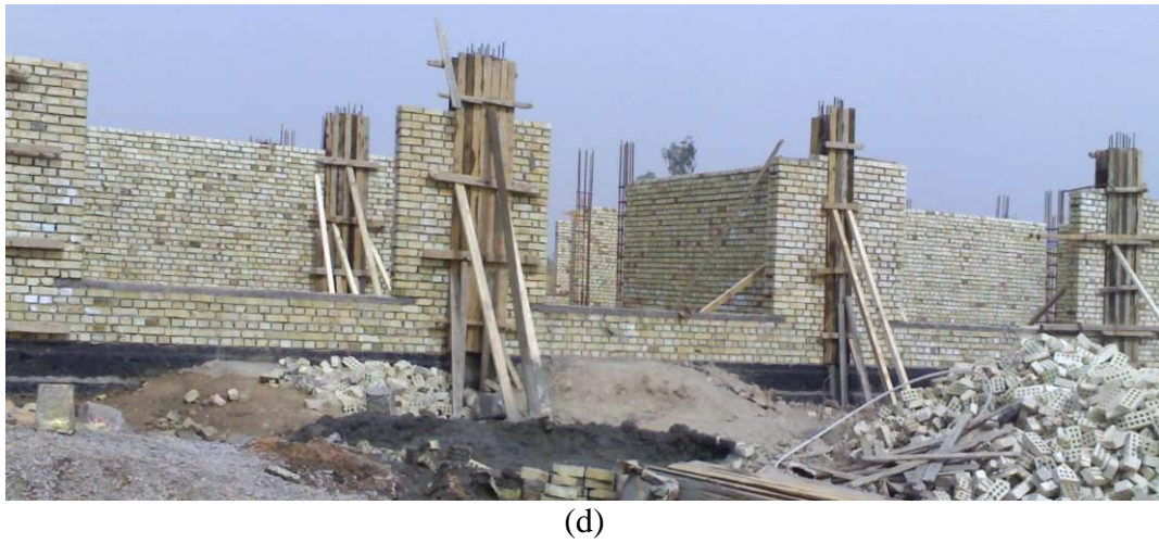
Fig (5): The building (D) was constructed by using tooth edge connection
