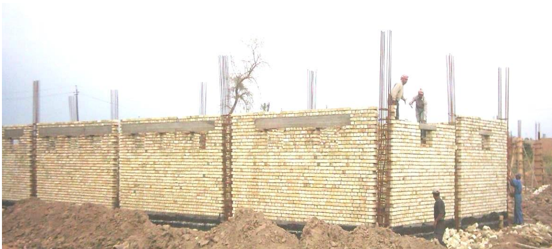
Fig. (1): The confined masonry building: (a) parts of building, (b) tie-column (tooth edge)
