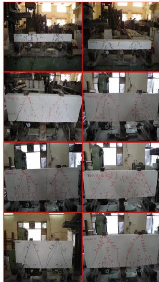
Figure 9: Cracking Patterns of the Tested Beams
