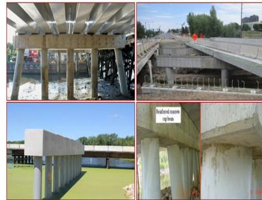
Figure 1: Pile Caps Behave as Continuous Deep Beams
