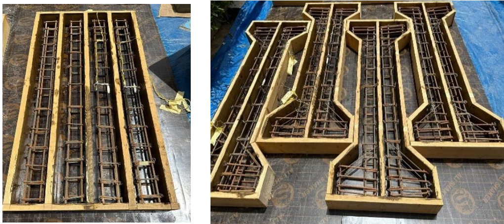
Figure 2. The wooden forms and reinforcement of concrete columns
