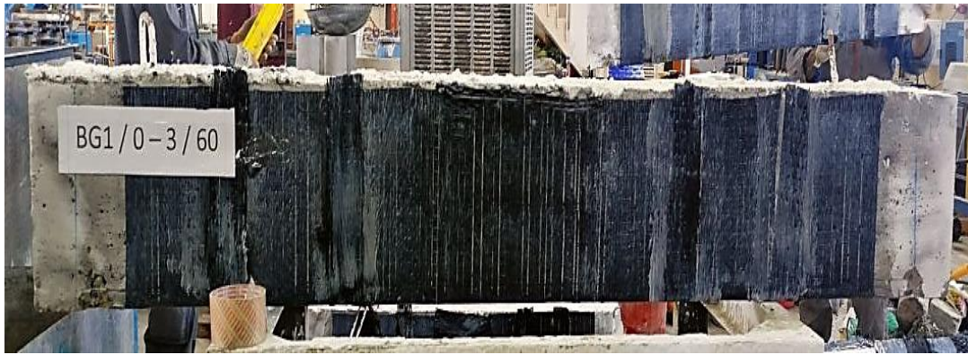
Figure 4. Beam after rehabilitation
